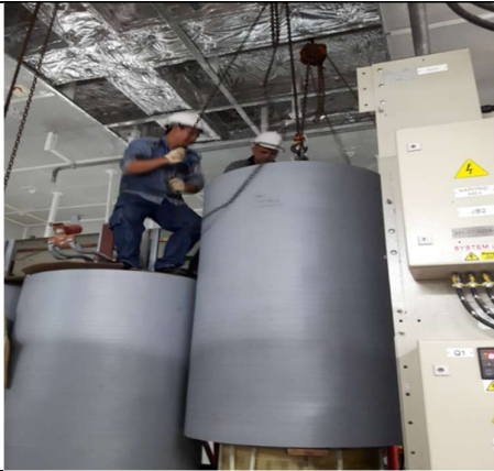
SỬA CHỮA MBA KHÔ 9500KVA – 6,3/0,4KV GIÀN KHOAN DẦU KHÍ LAM SƠN REPAIR OF DRY TRANSFORMER 9500KVA – 6.3/0.4KV LAM SON OIL AND GAS DRILLING RIG
