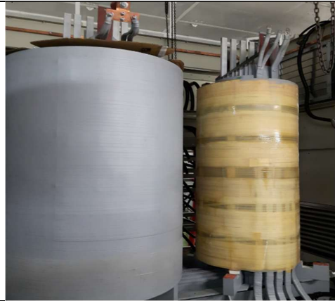
SỬA CHỮA MBA KHÔ 9500KVA – 6,3/0,4KV GIÀN KHOAN DẦU KHÍ LAM SƠN REPAIR OF DRY TRANSFORMER 9500KVA – 6.3/0.4KV LAM SON OIL AND GAS DRILLING RIG
